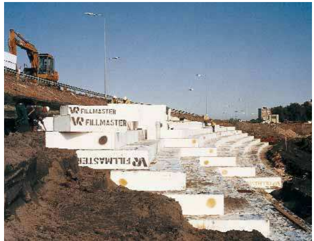
Work on the Priory Way spur road
